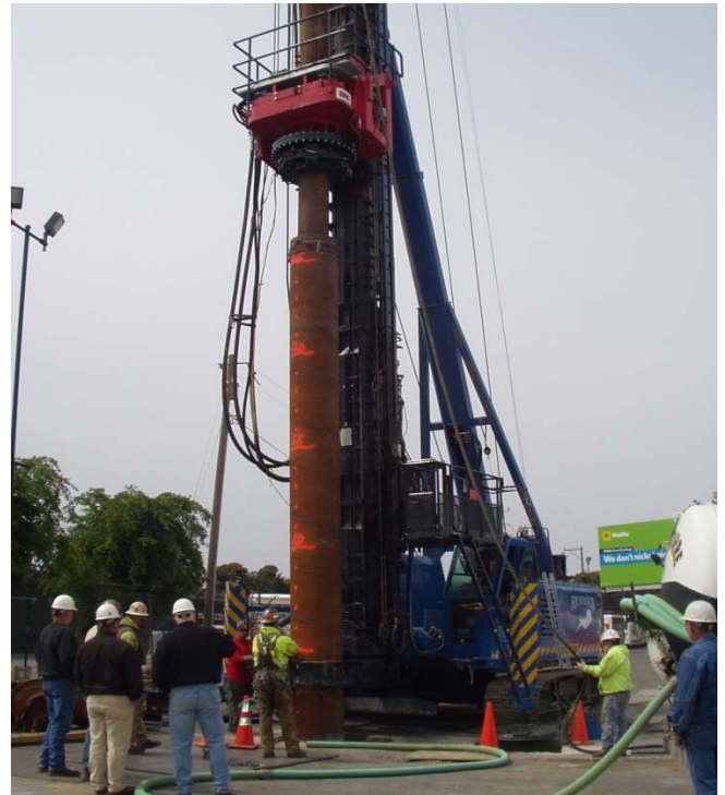
Clear Channel Sign Foundation 30" TGIP-San Francisco, CA
