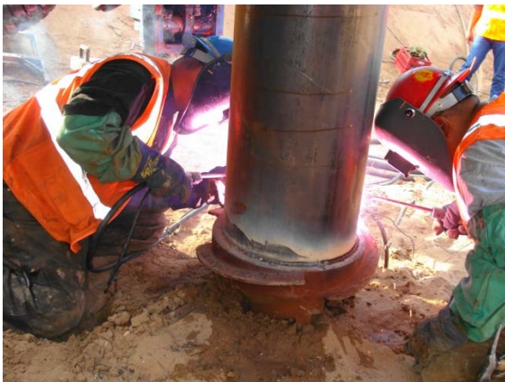
Sample Tip Installation Method Jeffery Road-Irvine, CA
